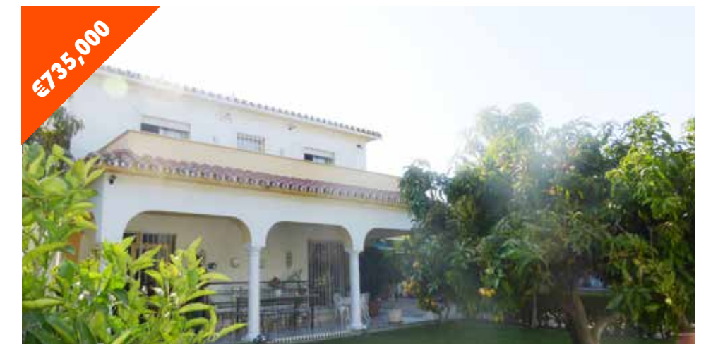
SAN PEDRO 4 Bed • 2,5 Bath • Built 233 m 2 • Ref KMSSP82 Great opportunity to modernise this lovely villa located only a few moments' walk from the beach, town and boulevard.
